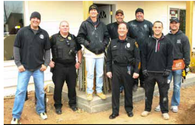
Prescott Valley Police Department volunteers traded their service weapons for nail guns to help the Prescott Area Habitat for Humanity "Build Homes & Build Hope."
